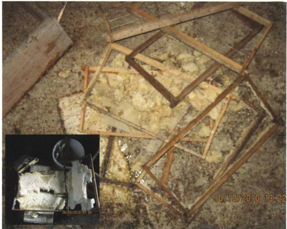
Shattered frames. Photos: Brian Lancaster.
